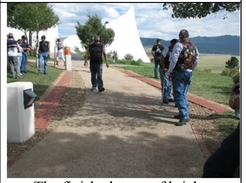
The finished rows of bricks
